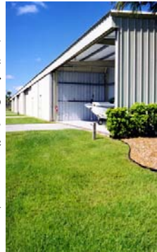
Typical T-Hangar at SEF
